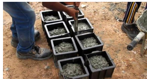
Compacting the concrete in the cube mould (For 150 mm cube at least 35 tamps per layer)
